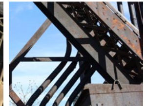
Train Bridge detail - Aka "Iron Curtain"
